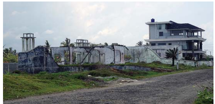
Fig. 7. Ruins around the only home standing after a 10-meter-high tsunami struck the coast of Java. The tsunami reached the upper floor of the three-story home in the distance.
